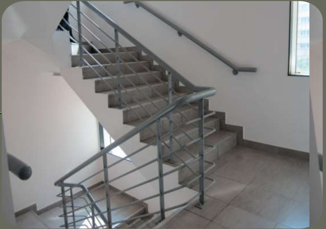
BOH Handrail at Reem Island
