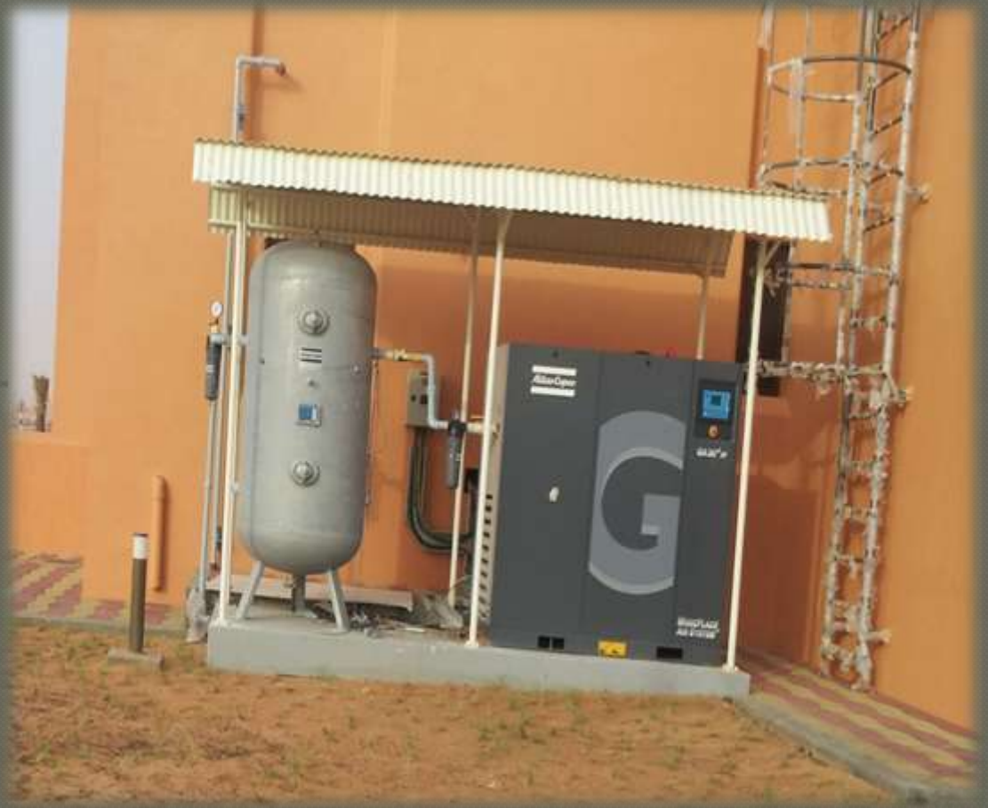
Compressor Shade for ADCO
