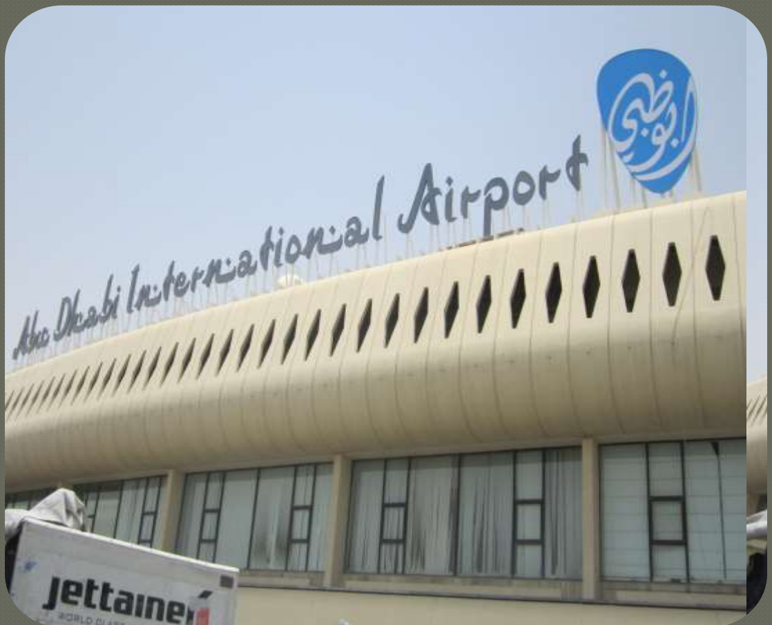
Abu Dhabi International Airport Sign board back Structure
