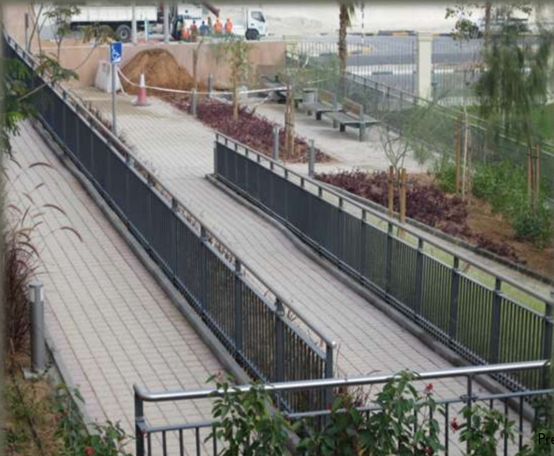
External Balustrade with top Rail at Sorbonne
