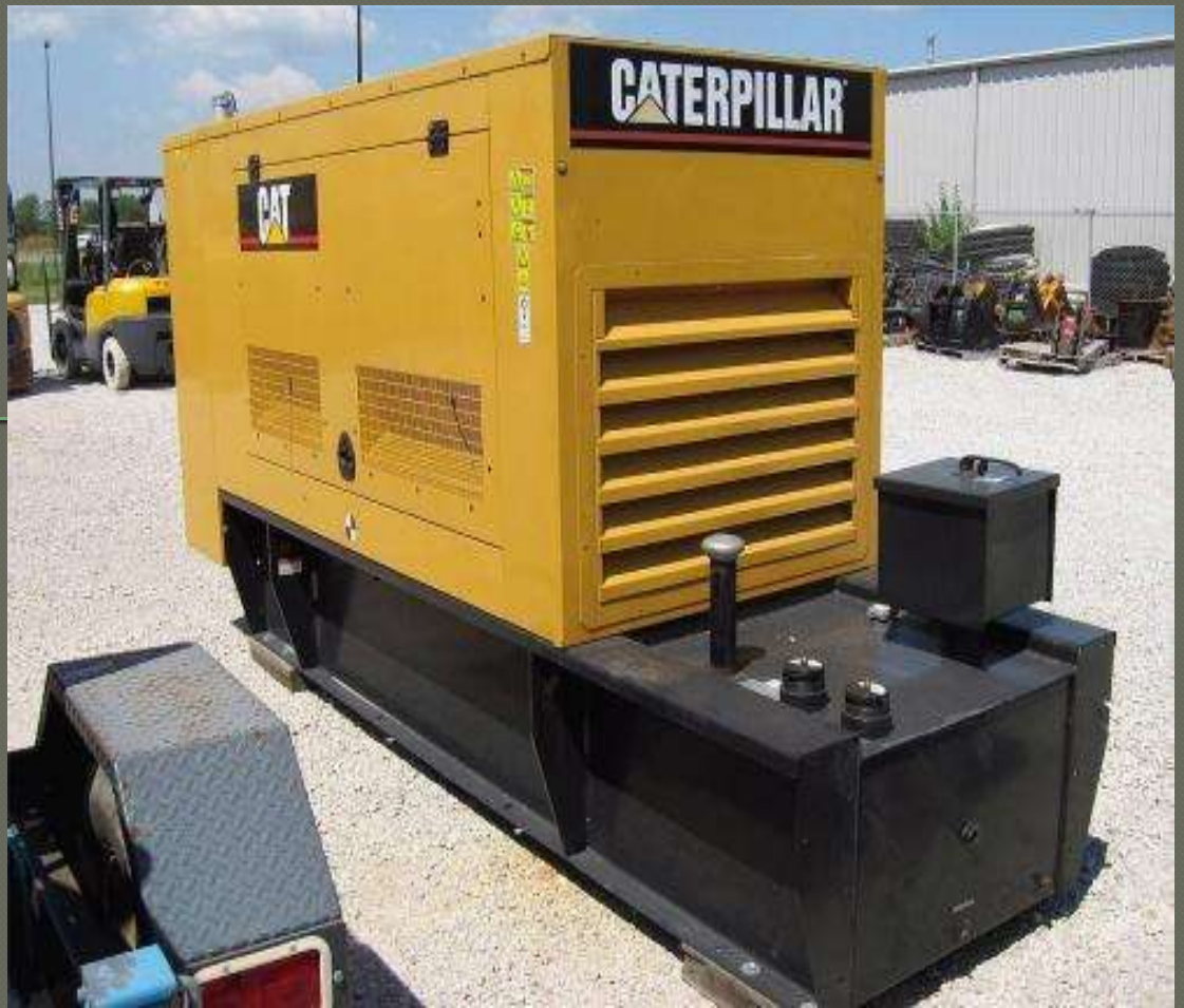
Base Tank for CAT Generator
