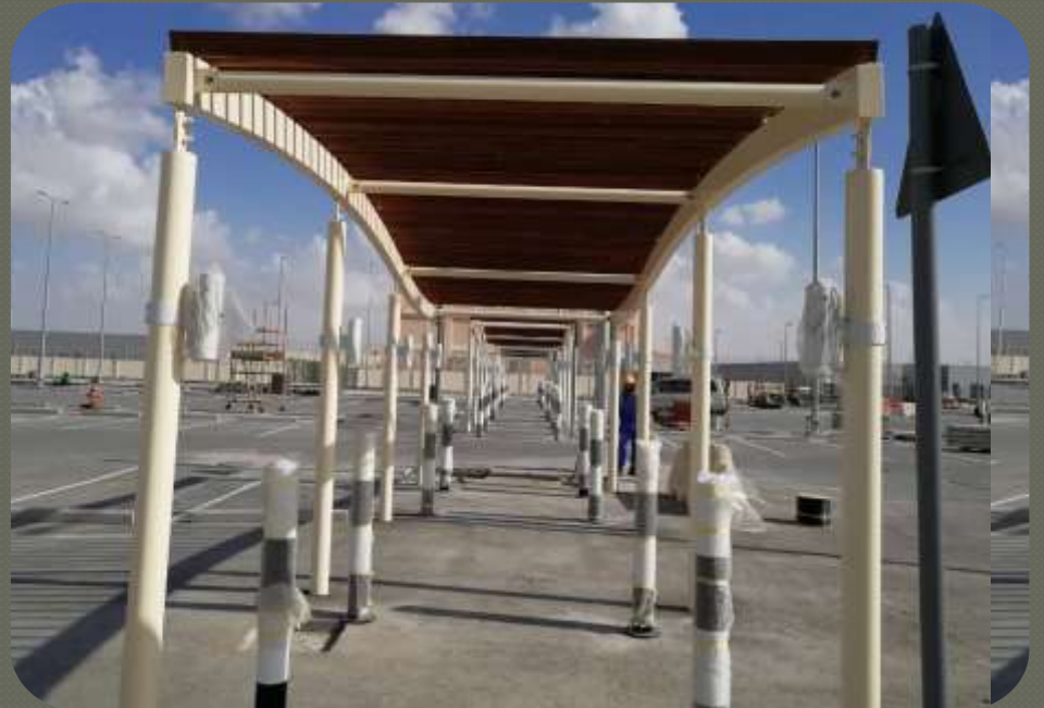
Shade Structure Midfield Terminal Abu Dhabi
