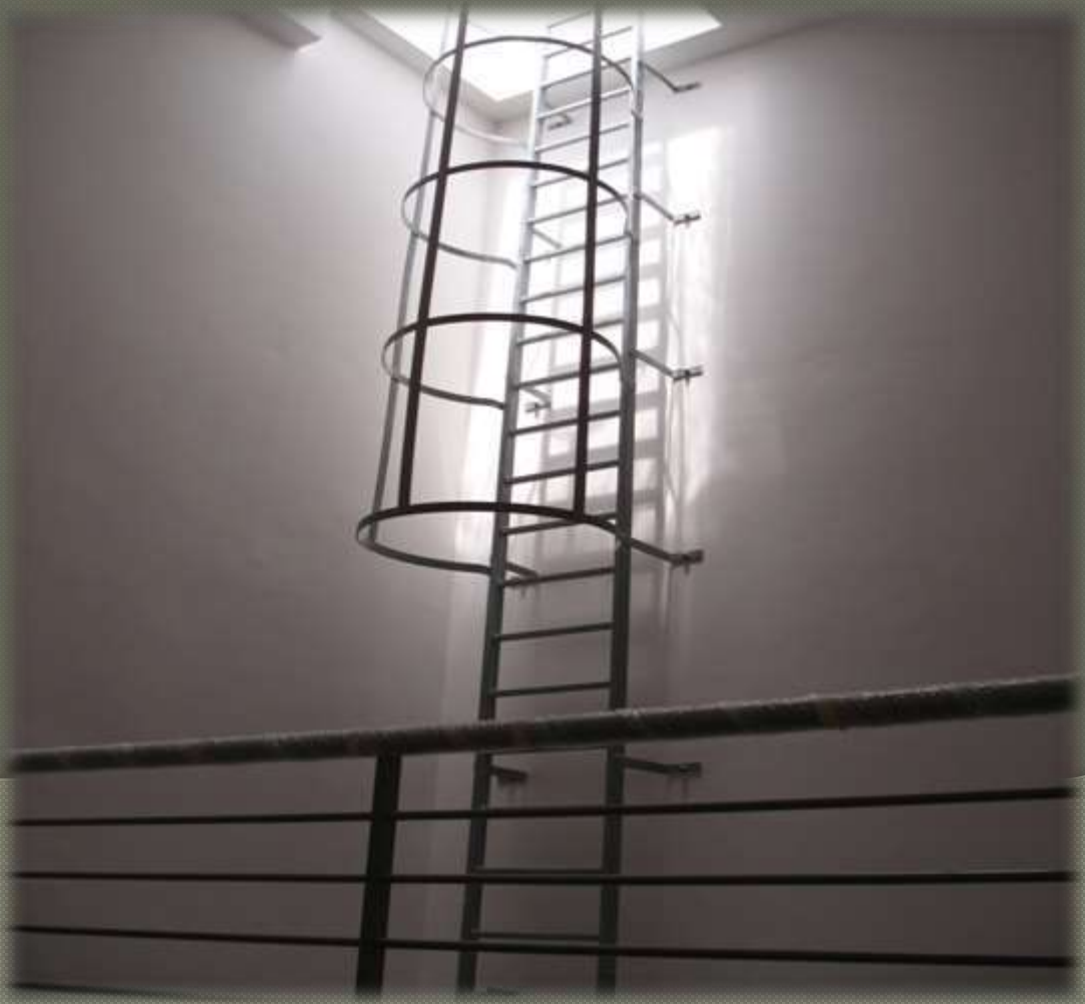
BOH handrail with Cat Ladder at Sorbonne University
