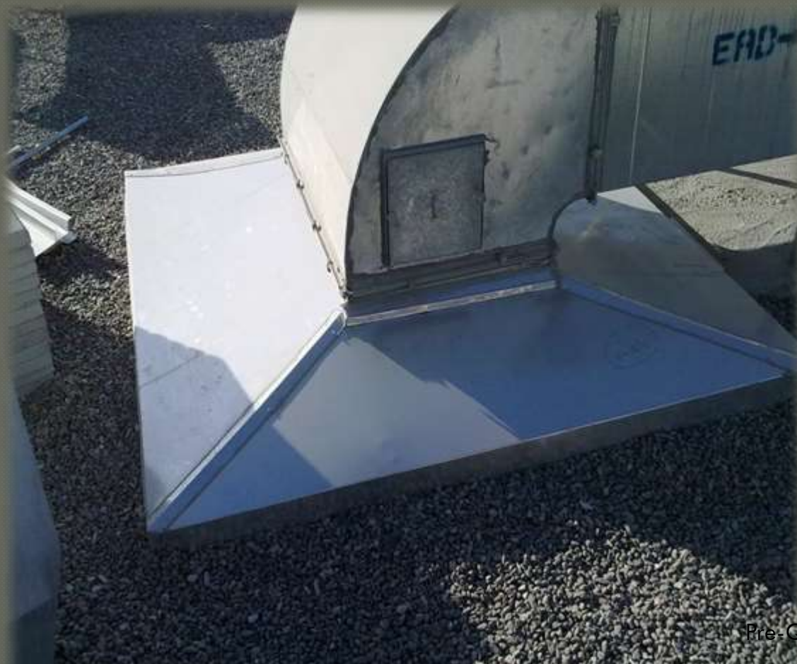
Aluminium flashing at AC Duct at Sorbonne University
