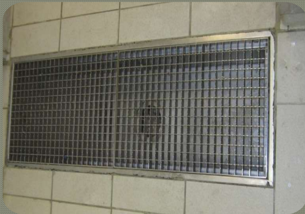
Stainless Steel Grating St. Regis Hotel at Sadiyat Island
