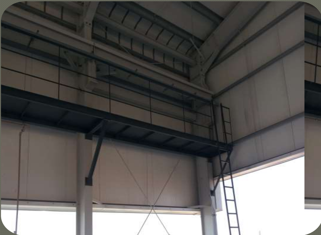
Metal Platform With Ladder for ADCO
